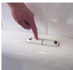
If you have dual-flush already fitted in the cistern, use the half-flush (3 litres) whenever appropriate. It saves many litres a week.
