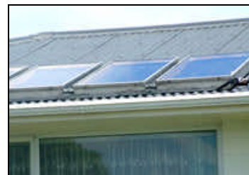
Solar water-heating panels can be metal or plastic, fitted onto or into the roof, and are usually glass-glazed, over either a black heat plate or a set of parallel glass tubes.
